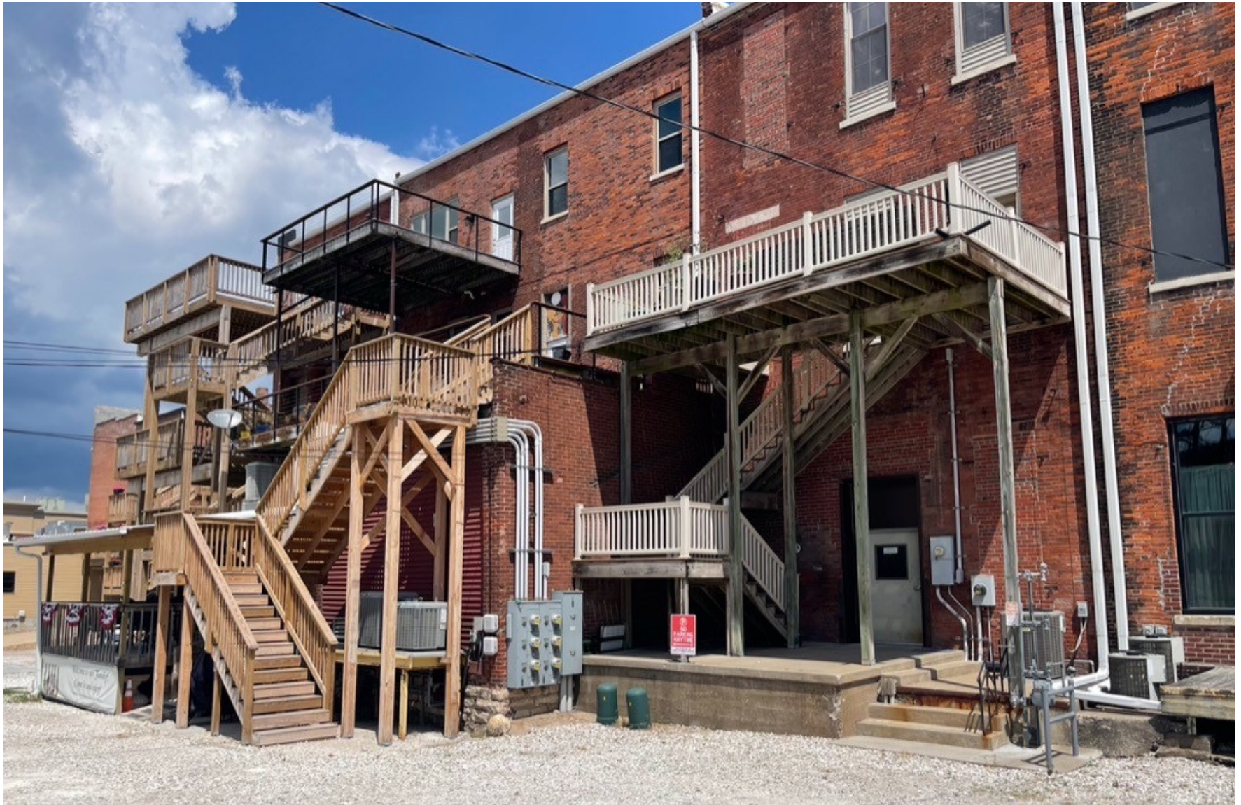
Area of refuge balcony added to the rear
